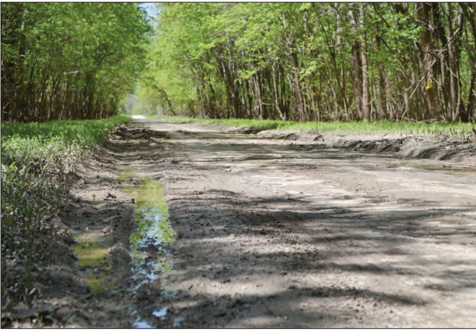
PHOTO BY DARYL K. TABOR/THE PRESS E-Town Ferry Road in northern Crittenden County has recently emerged from a second round of Ohio River backwater this year. Each time the river floods, silt and debris deposits build up the land on either side of the 1.2-mile road, leaving mud and water no place to drain, burying the surface under the muck. Last week, a federal disaster declaration could make the county eligible for reimbursement to alleviate problems like this caused by late-winter flooding.
